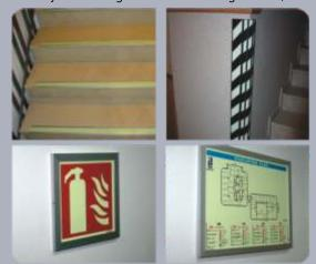
new frames for signs and emergency plans; the **③Everlux**° safety bumpers to give protection in case of collision and the **④Everlux**° step protection to protect the face of the steps.
