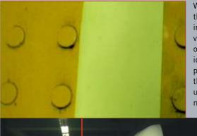
With this system the edges of the platforms can be marked in a way that allows the visually impaired and all other passengers to easily identify the edges of the platforms which increases the comfort and safety of all users of the underground rail network.
